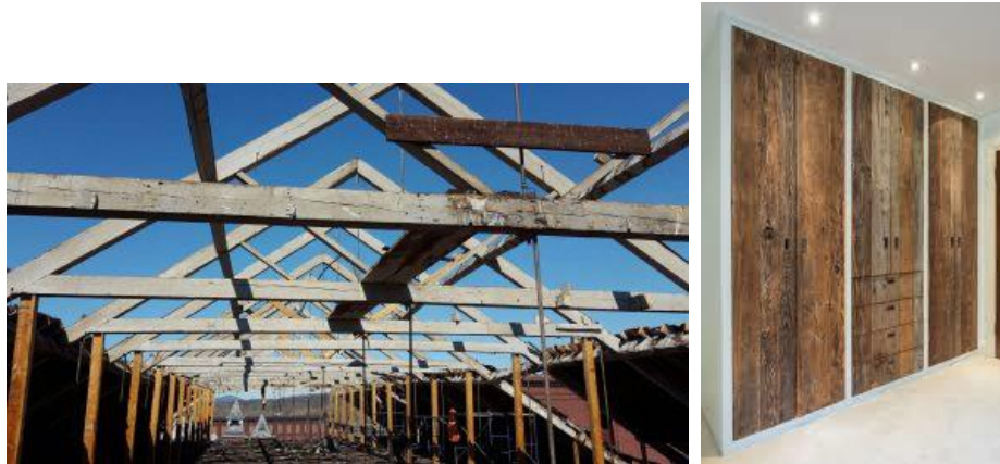
Figure 17: Reused wood framing and panels
