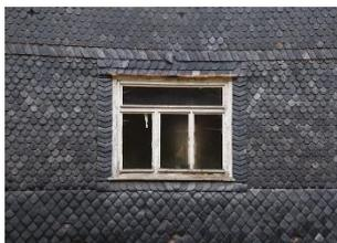
Figure 19 Slate shingles as wall finishing in historic buildings
